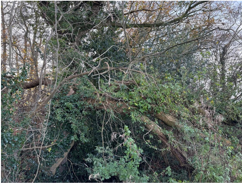
Photograph 3 A veteran common oak (T13) located at the northern end of the ancient woodland. Partially collapsed towards the Construction and Operation Area with significant decay in collapsed sections.
